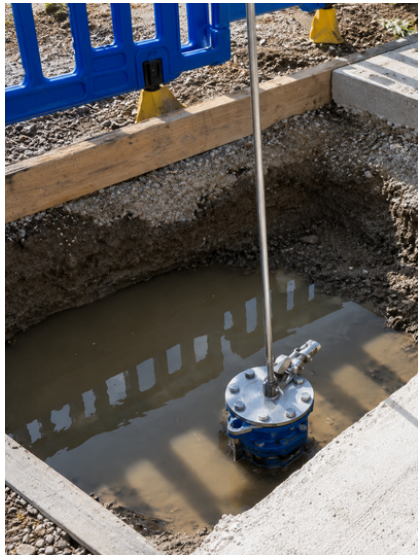
Insertion of the Nautilus sphere using non-invasive systems
