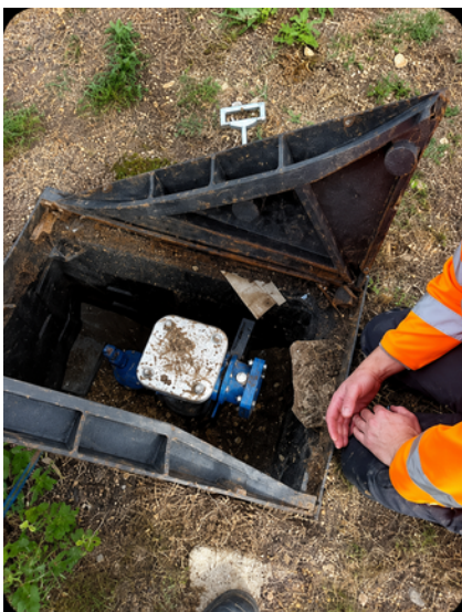
Installation of synchronizers along the pipeline.
