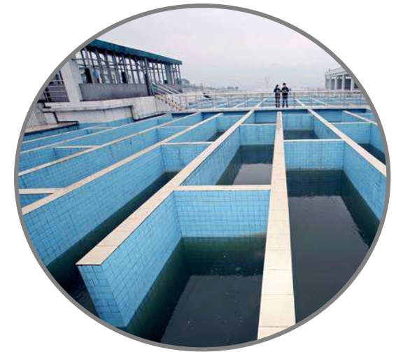
Water treatment plant in France
