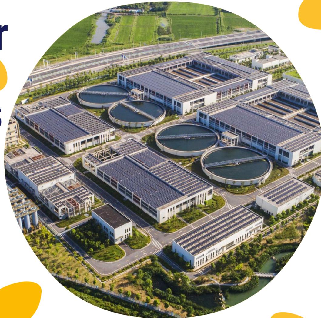
Spanning around 90 hectares and with a total capacity of 120,000 m<sup>3</sup>/day, the wastewater treatment plant (WWTP) serves a population of 461,400. The plant uses 30% of the recycled water in various ways, in particular to irrigate green spaces and roads.
