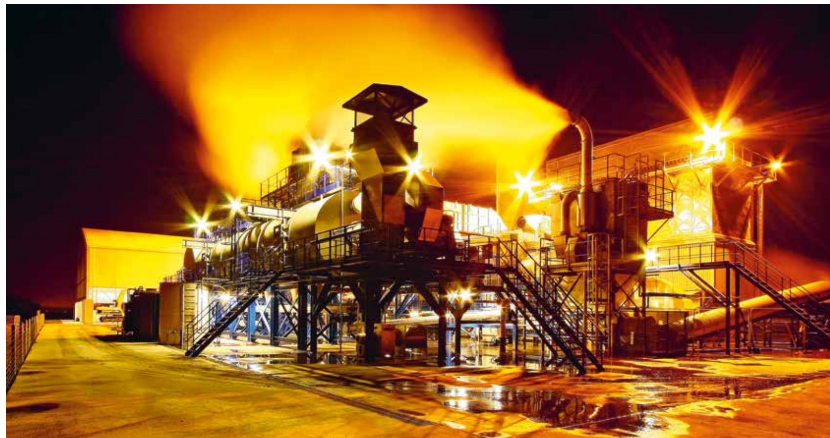
Rehabilitation of The Avenue coking works in Chesterfield, England
