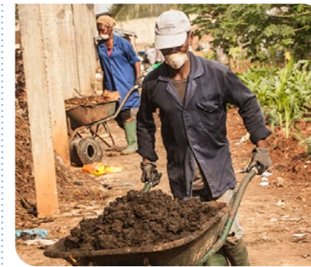
A recovery project reference in Africa
