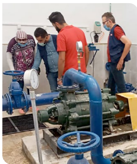
Reestablishing and reinforcing infrastructures
