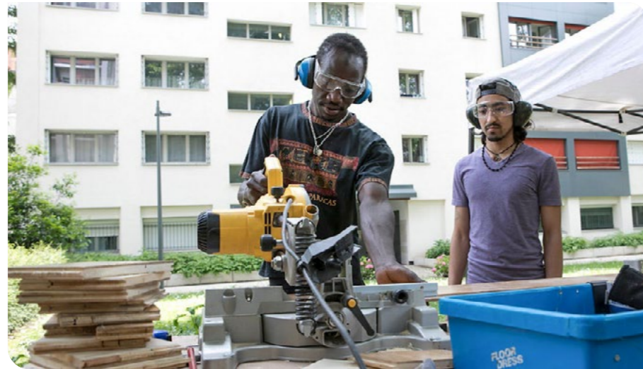
Training to become “carpenters within a circular economy”
