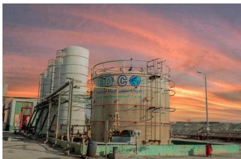
© EDCO plant in Saudi Arabia / SUEZ.
