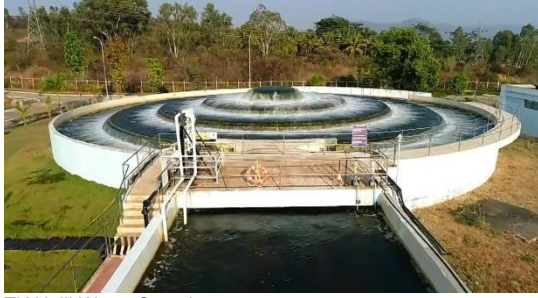
TK Halli Water Complex
