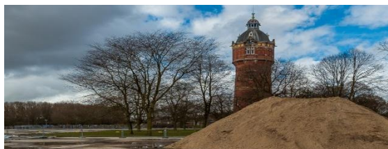
The former industrial district of Amstelkwartier is to be rehabilitated and depolluted. Amstelkwartier, Amsterdam (Netherlands) ©SUEZ
