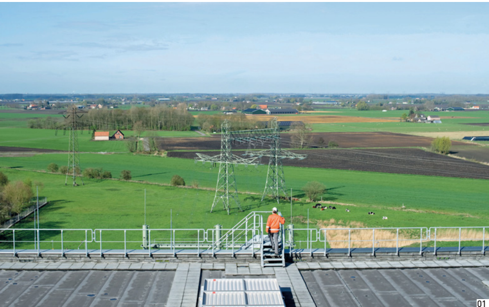
01_ Connected to the electricity grid, ReEnergy generates 256,000 MWh of electricity.
